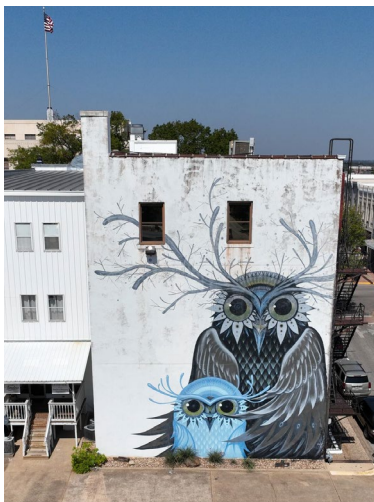
Existing Conditions, Rear Facade
